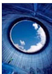
Cover photo: Terminal for liquid natural gas in Nynäshamn, Sweden. Photo: Bruno Ehrns.
